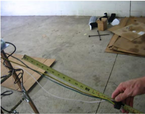
Pull the excess wire out of the back of the tongue section leaving approximately 18" of harness exposed at the front.
