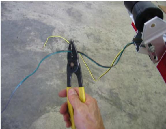
Cut the excess wire at the rear of the trailer leaving 12" exposed.
